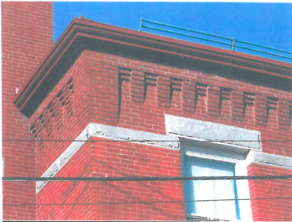
Decorative Dentil Corbelling at South Elevation of the Original 1888 Building
