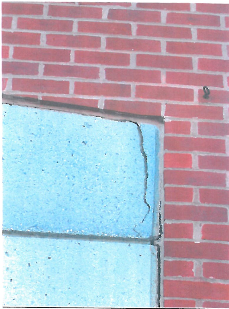
Cracking and Separation at Precast Lintel of the 1988 Addition
