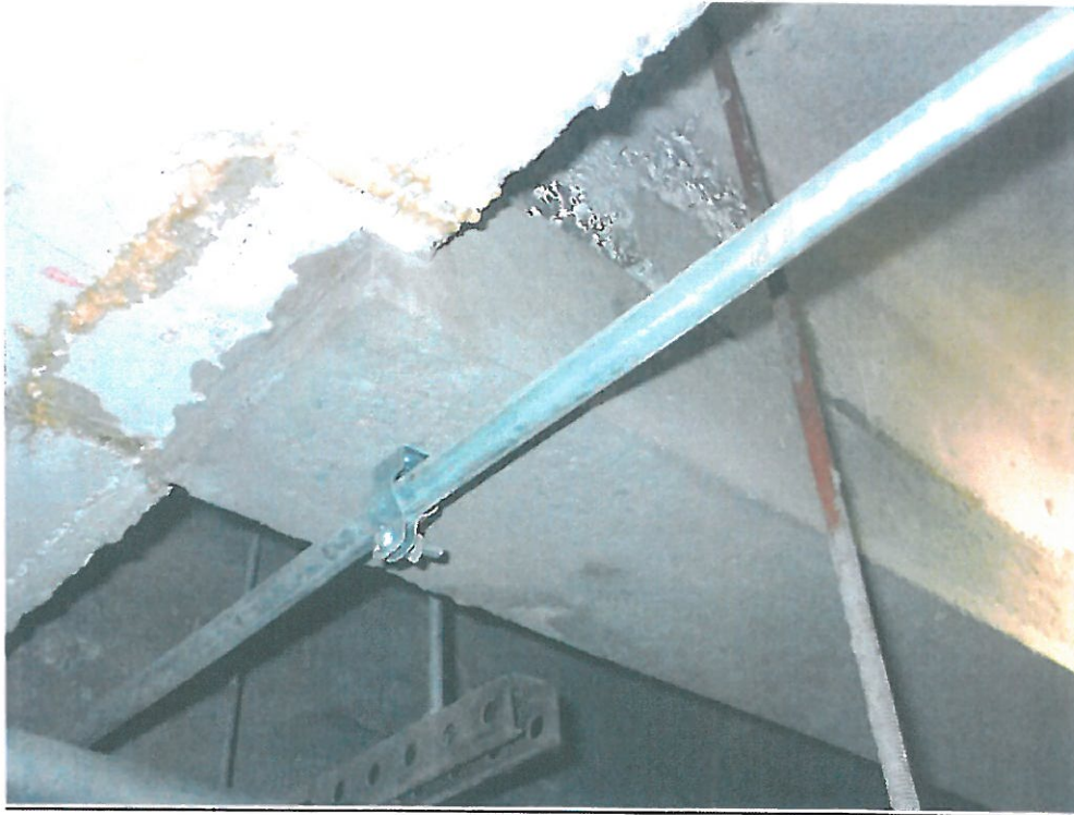
Repairs to Underside of Floor Structure
